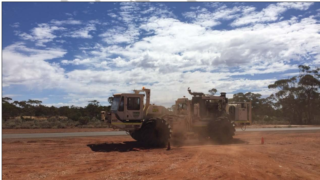
Figure 8: Renegade seismic vibrator in action in the Eastern Goldfields. These 80,000 lb units, operated by Velseis, are the most powerful seismic sources available in Australia and provide superior deep stratigraphic images.
