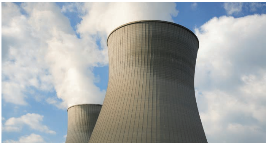
Traditional nuclear energy generation and new small modular reactors (SMRs) are part of the low carbon mix. EnE is providing environmental services for license renewal of operating reactors—including Callaway and Braidwood—and licensing of the proposed Fermi 3 nuclear power plant.
