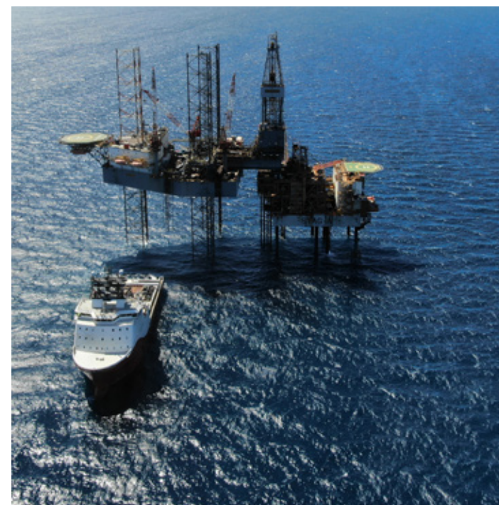
Jack Up rig Enasco 107 operating over the Stag Platform
