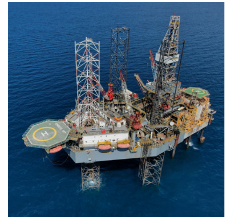
Enssco 107 drilling rig and Stag platform
