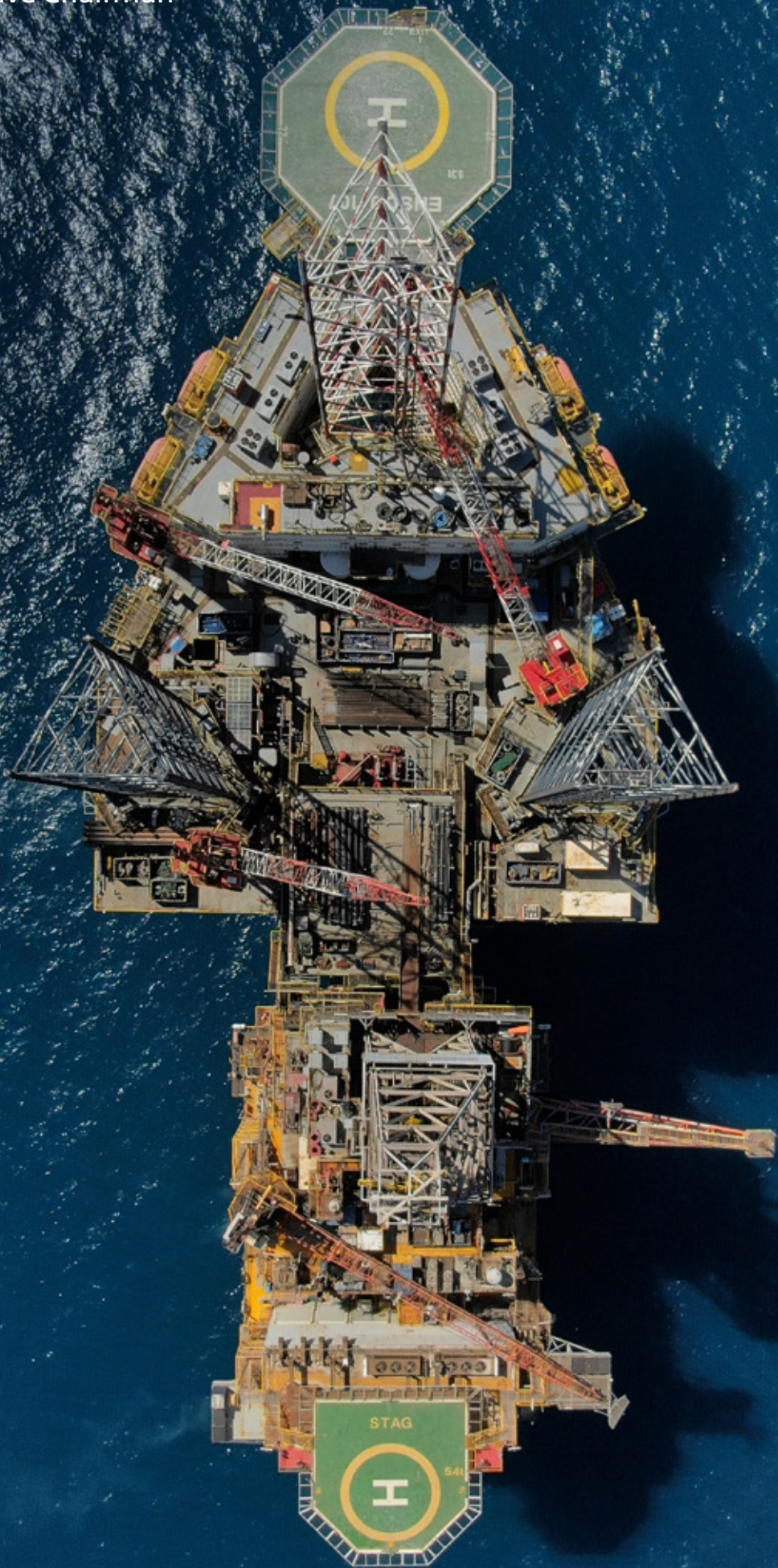
Stag platform with the Ensko 107 drilling rig
