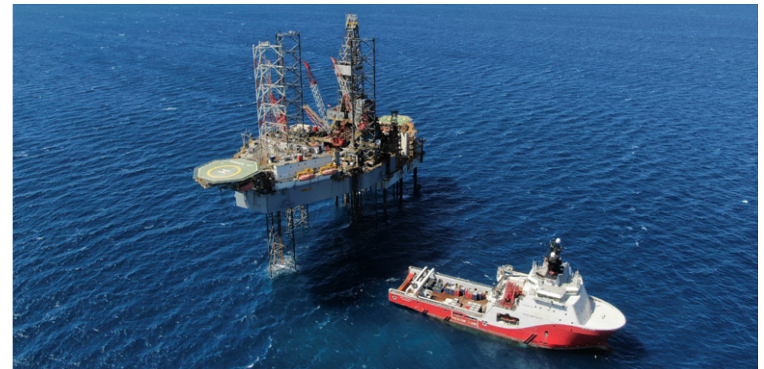
Stag platform, Ensco 107 drilling rig and support vessel
