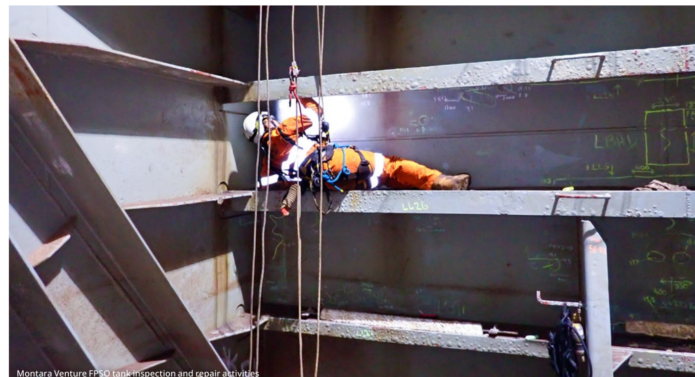
Montara Venture FPSO tank inspection and repair activities
