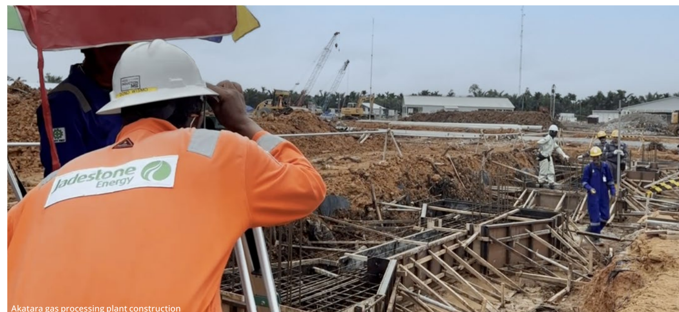
Akatara gas processing plant construction
