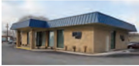
The newly-remodeled Orchard Park office.
