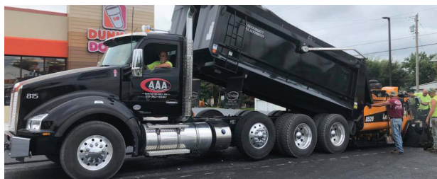
Photo provided by AAA Paving & Excavating Inc.
