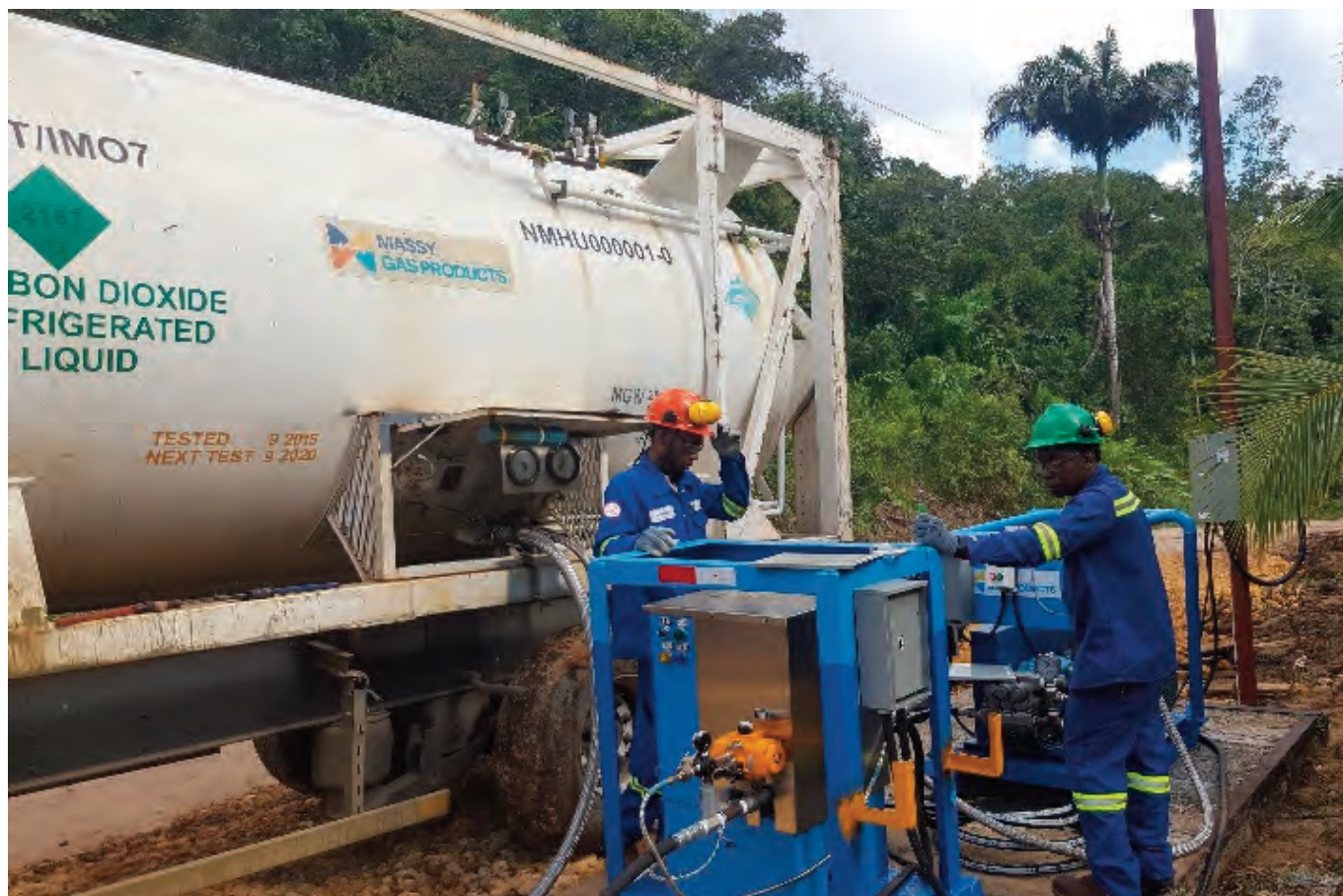
CO2 being hooked-up for injection
