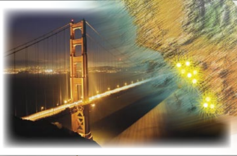
Golden Gate Bridge, San Francisco
