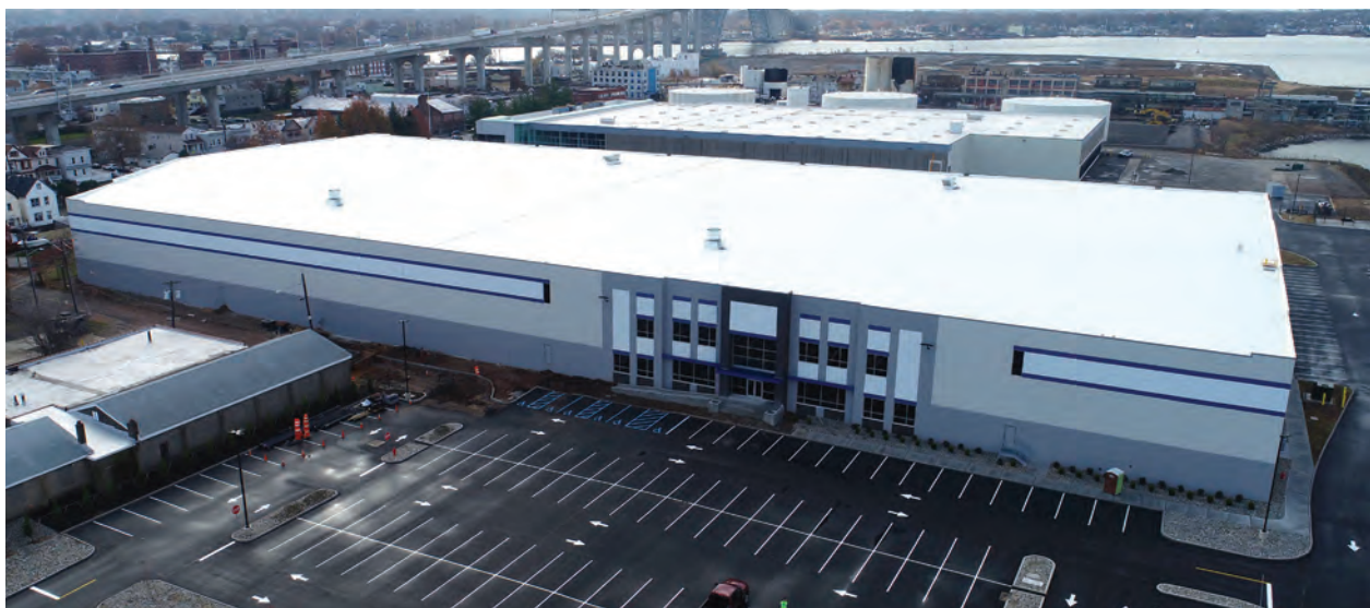
Properties located at 99 and 105 Avenue A, Bayonne, New Jersey.
