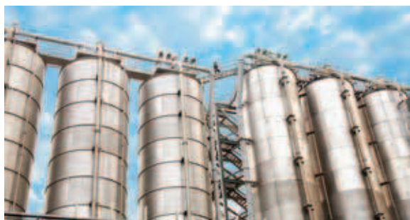
PP Plant at Jamnagar
