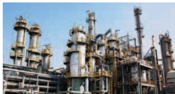
Methyl Ethylene Glycol plant at Hazira
