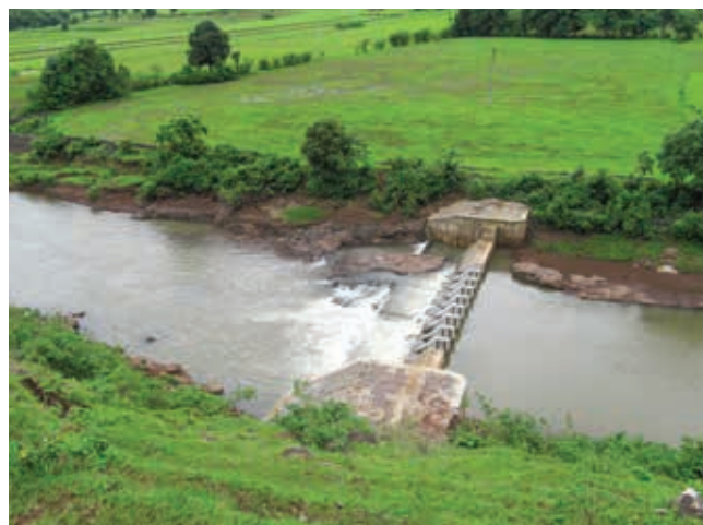
Water conservation in a check dam at Moyari, Chhindwara, Madhya Pradesh
