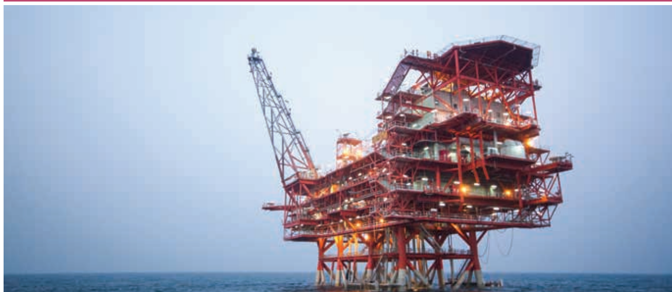
Control riser platform KG D6
