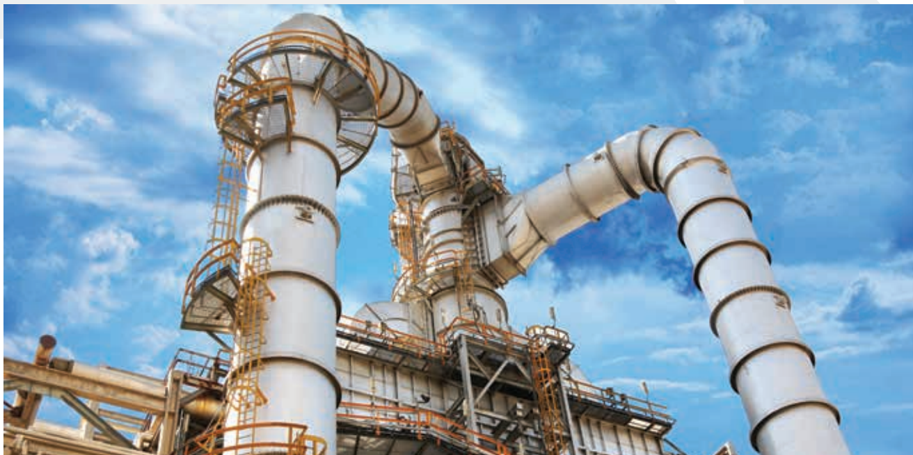
Heater of Aromatics Complex at Jamnagar Refinery
