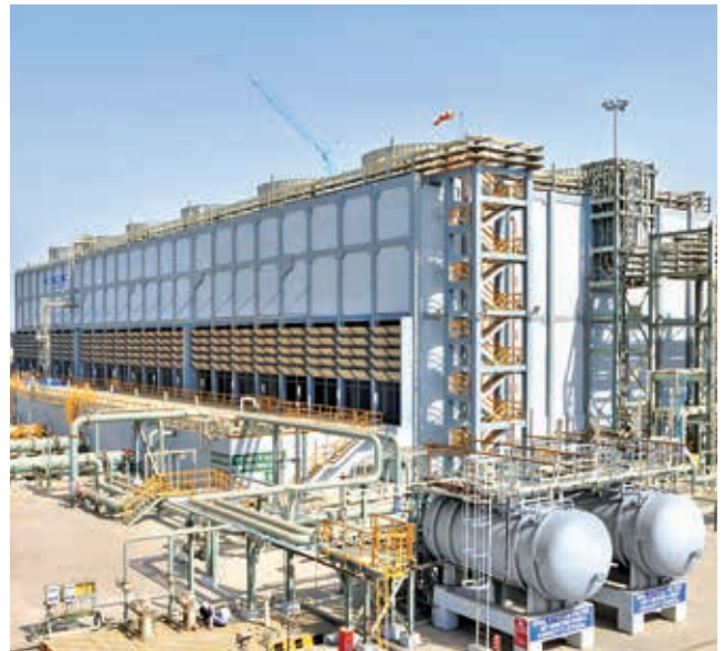
Gasifier-Cooling Tower
