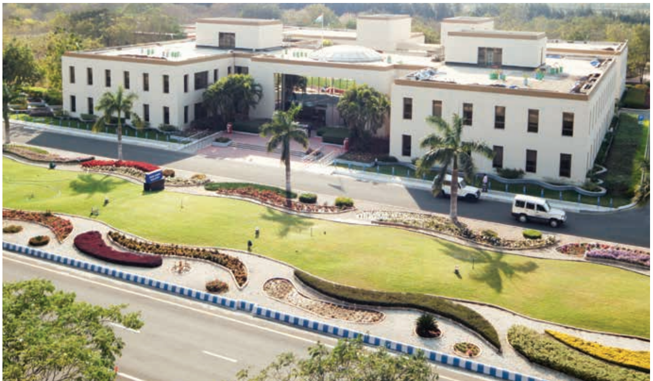
Jamnagar admin block
