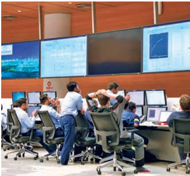
Gasifier Control Centre
