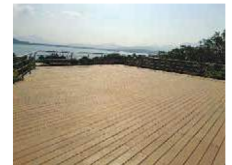
Relwood used for outdoor decks
