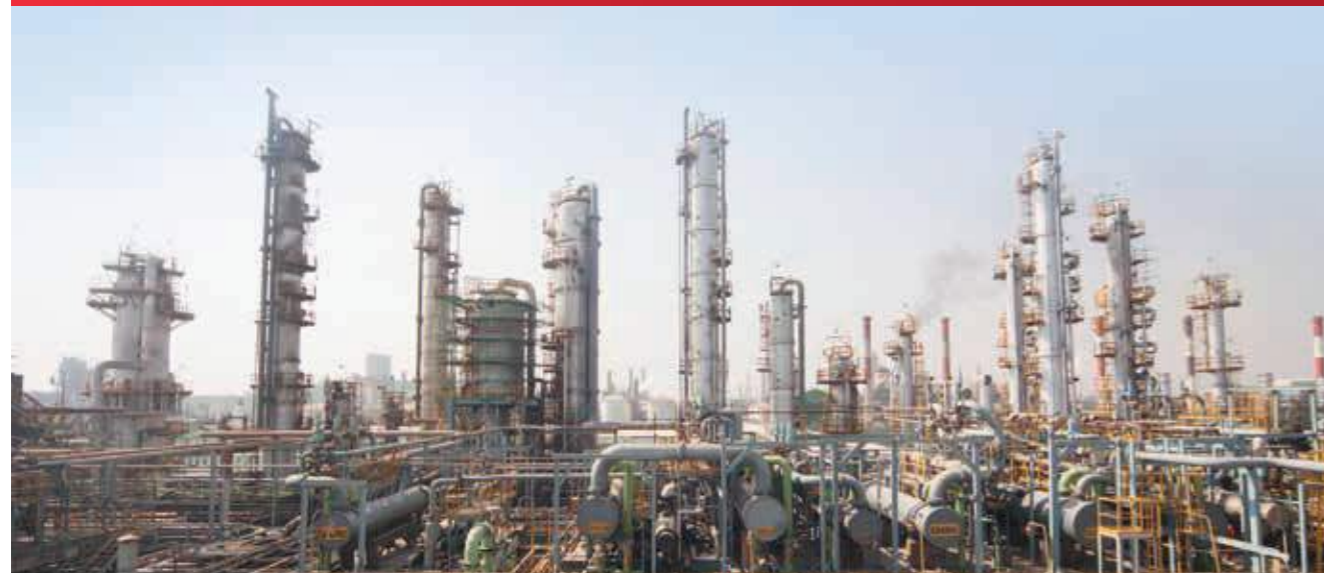
World-class production facilities
