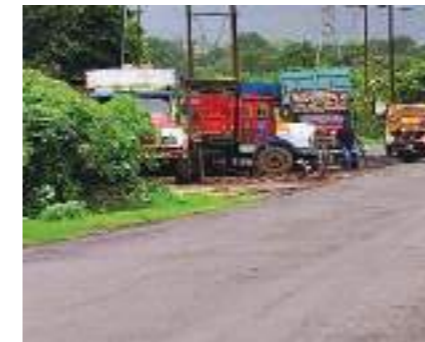
High quality of ReRoute roads even after monsoons
