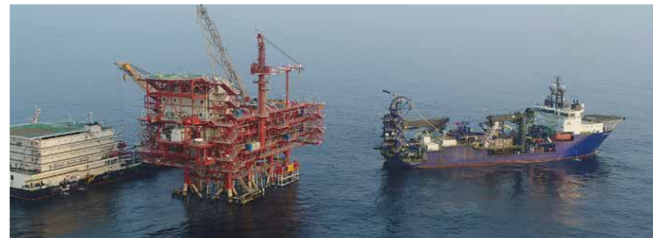
CRP modifications underway
