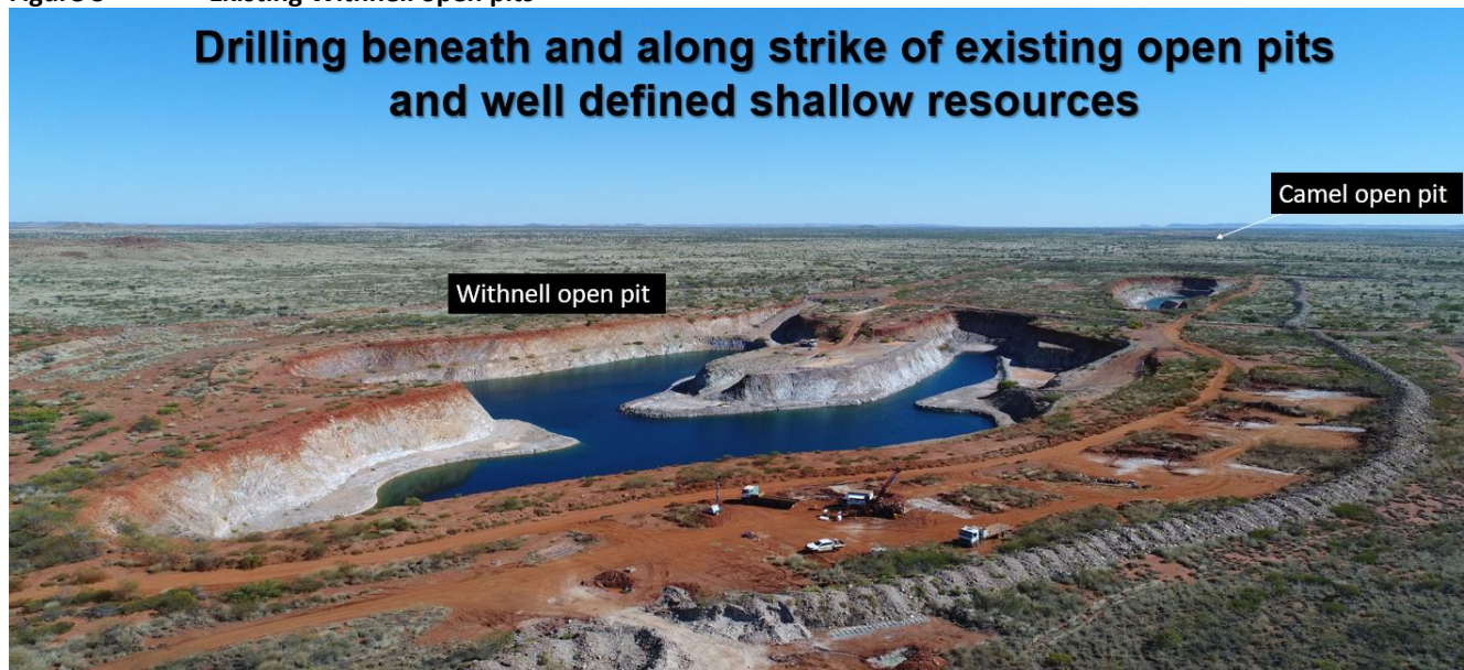
Figure 3 Existing Withnell open pits
