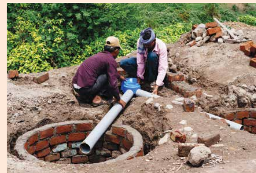
The SATO V-Trap is designed to reduce the risk of pipes becoming clogged with excrement. In addition, whereas older systems required extensive work (including concrete removal, etc.) in order to install the junction box that allowed switching between pits, with the SATO V-Trap switching between pits can be accomplished easily using just a wooden stick.
