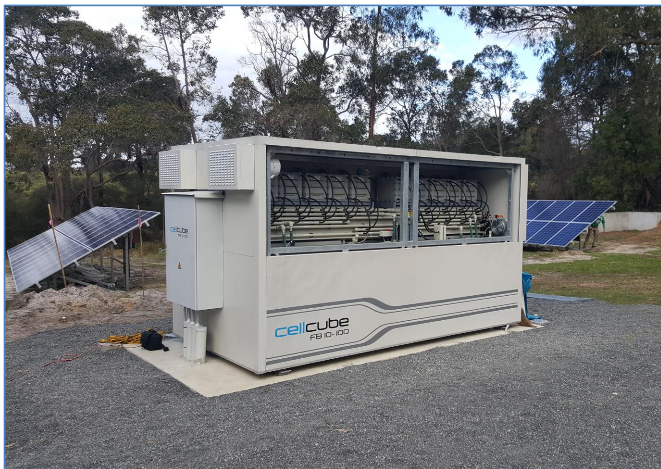
Figure 5: CellCube VRFB System on site at Busselton, Western Australia
